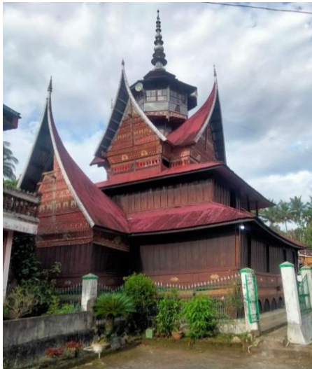
Gambar 1. Bangunan surau lubuk bauk (Ahmad Ash Shidiq, 2022)
